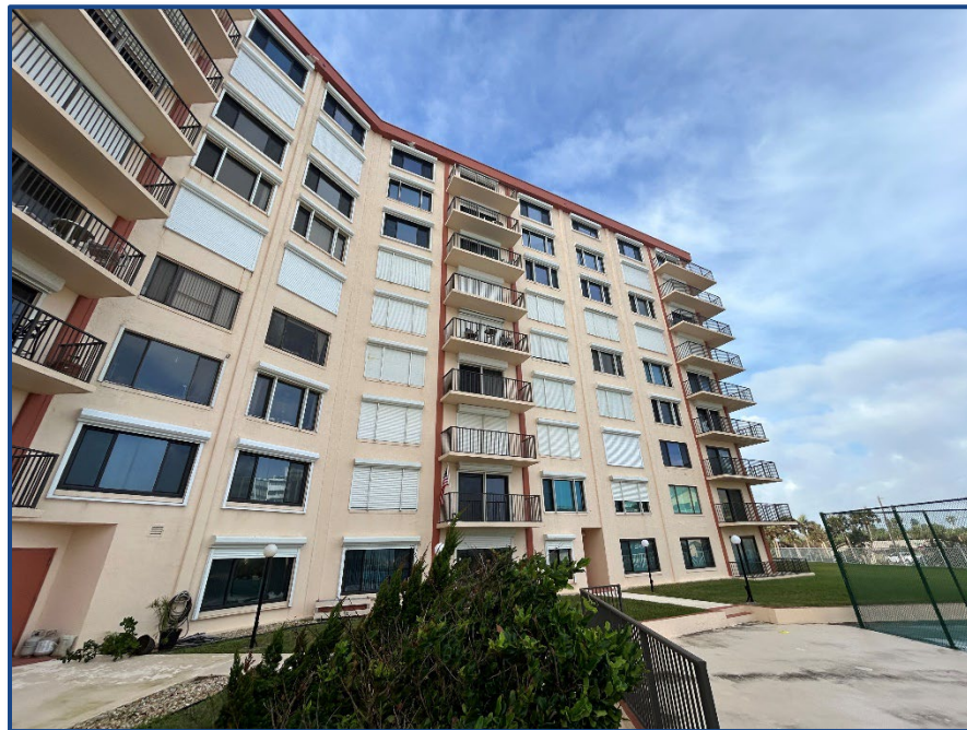
Photograph No. 6: Northeastern elevation.
