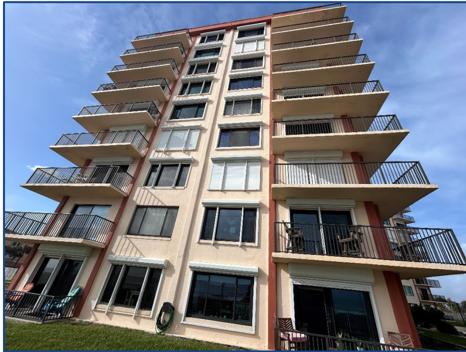
Photograph No. 4: Eastern elevation.
