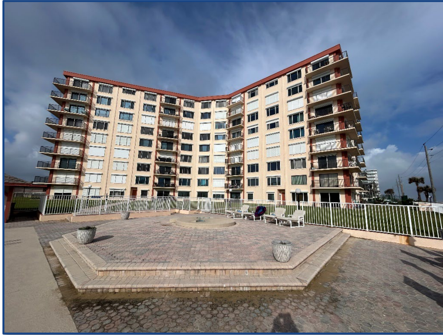
Photograph No. 3: Eastern elevation.
