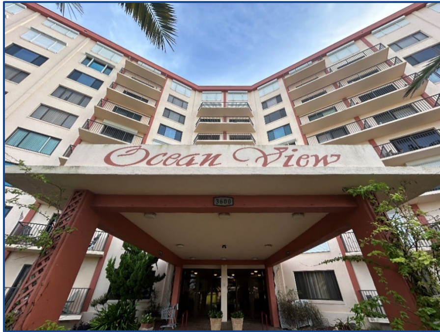
Photograph No. 1: Porte Cochere and building entrance located at the west side of the building.
