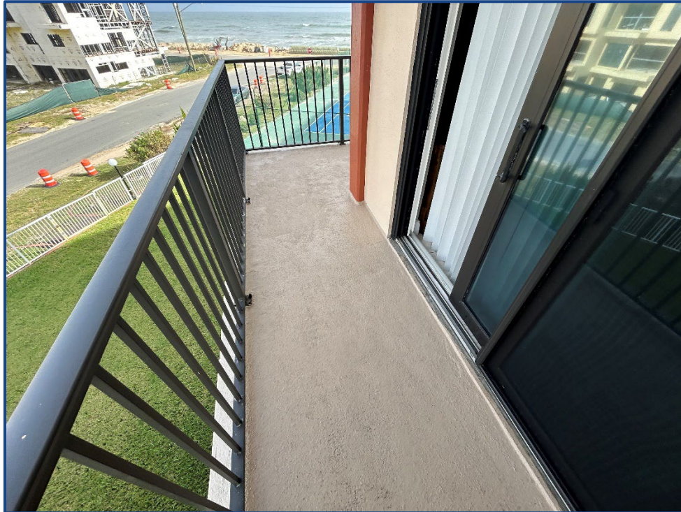
Photograph No. 40: Room 311 balcony area.
