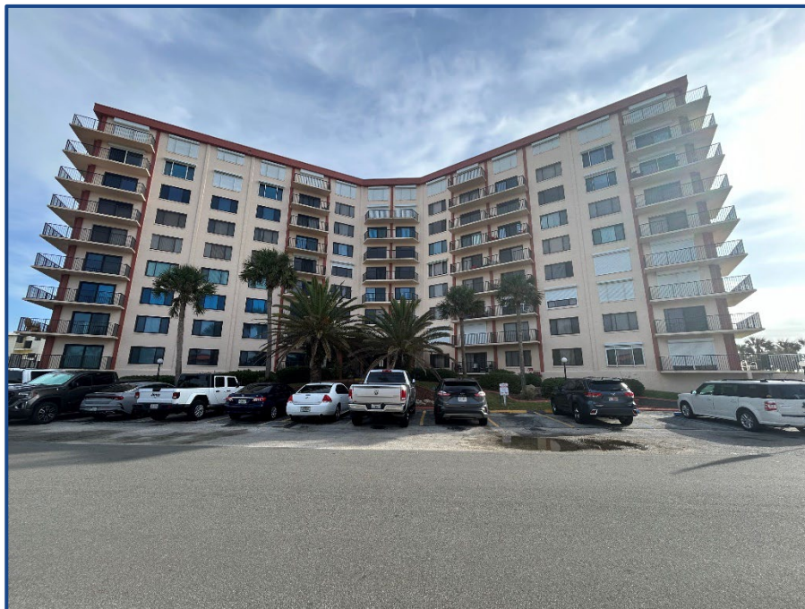
Photograph No. 2: Western elevation.
