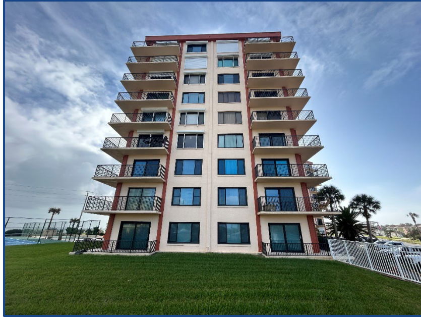
Photograph No. 5: Northwest elevation.
