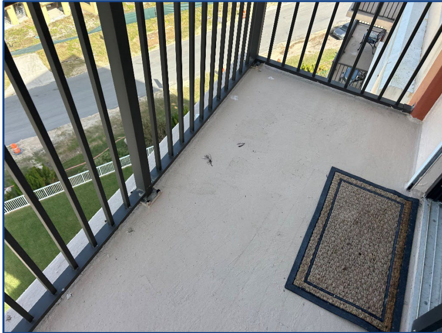
Photograph No. 50: Room 912 balcony area in good overall condition.
