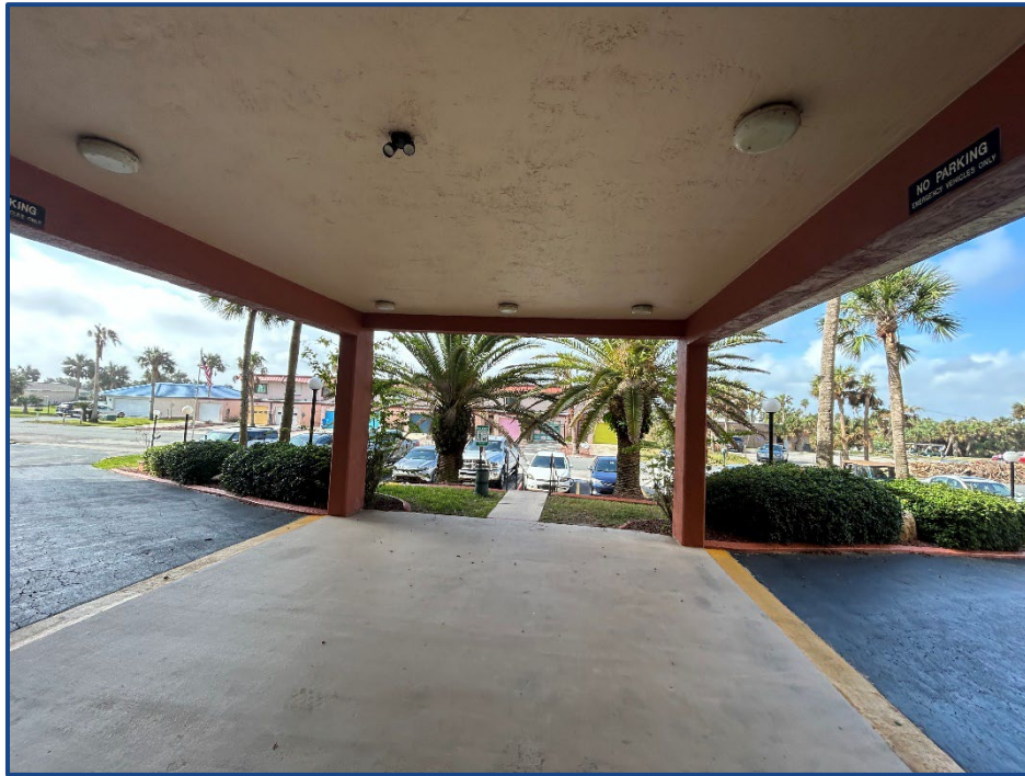
Photograph No. 37: Porte cochere located at the building entrance
