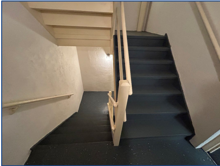
Photograph No. 29: Typical interior stairwell with metal stairs and aluminum railings.
