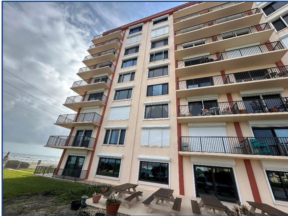
Photograph No. 7: Northeastern elevation.
