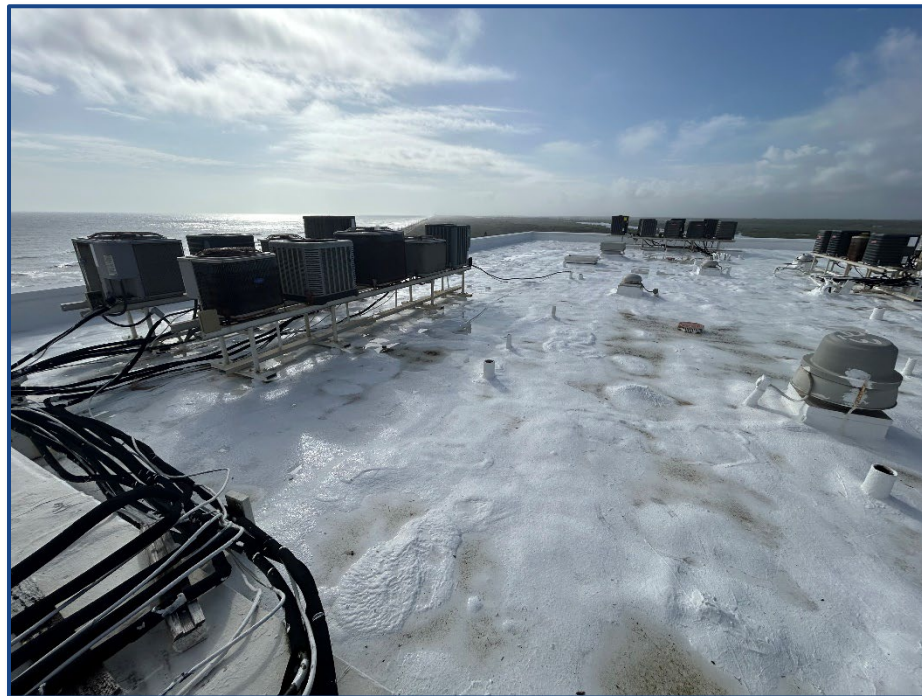
Photograph No. 14: Overall roof at the east wing of the building.
