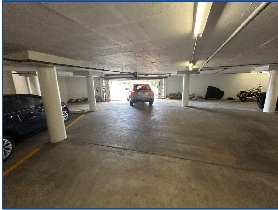
Photograph No. 11: Bottom floor garage door at entrance.
