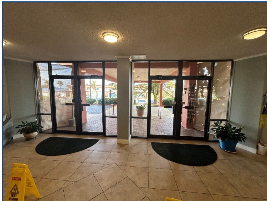
Photograph No. 8: Building entrance glass storefront.
