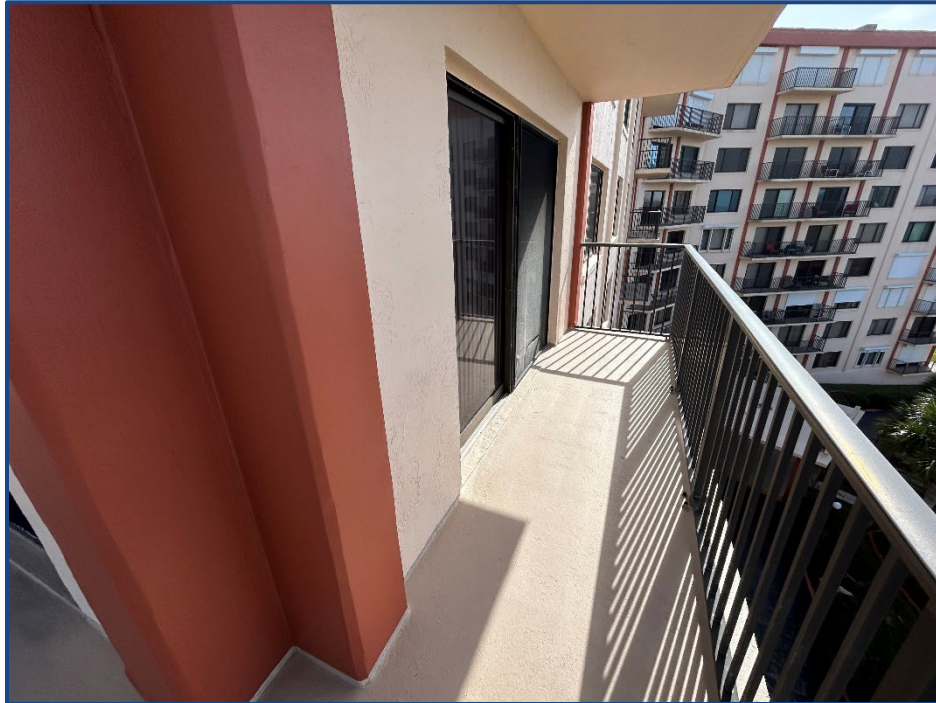
Photograph No. 48: Room 724 typical balcony area in good condition.
