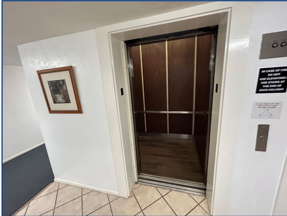
Photograph No. 28: Typical elevator door opening.
