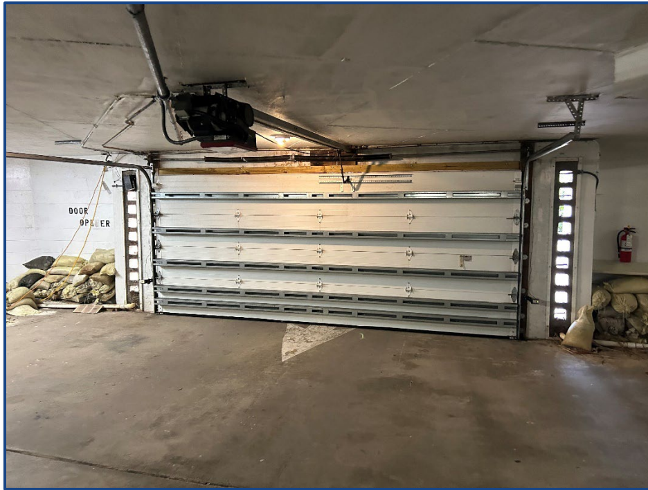
Photograph No. 25: Typical garage door located at the garage entrance.
