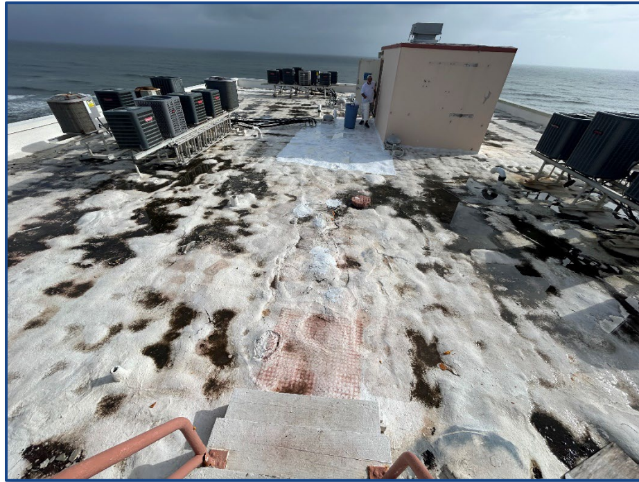
Photograph No. 13: Overall roof of the east wing of the building.
