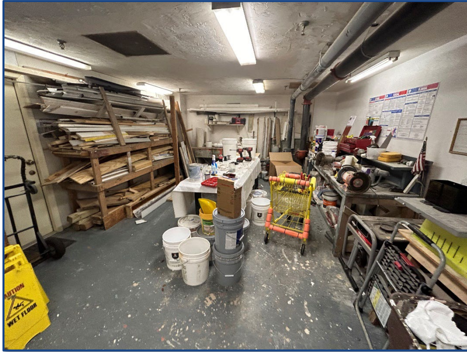
Photograph No. 27: Overall maintenance storage room.
